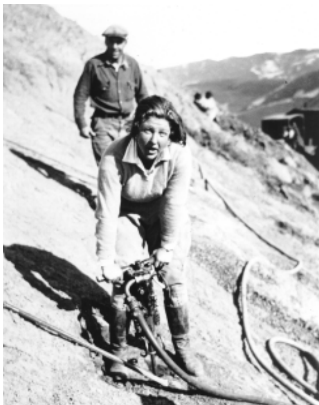
Figure 2. Laura “Dusty” Vail, daughter of William Banning Vail, preparing blasting holes for the roadway construction to Vail Peak in 1932.
